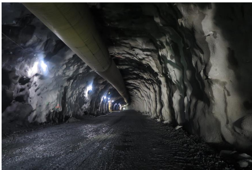
Figure 6. An under-construction road tunnel supported by systematic bolting and fiber reinforced shotcrete.
